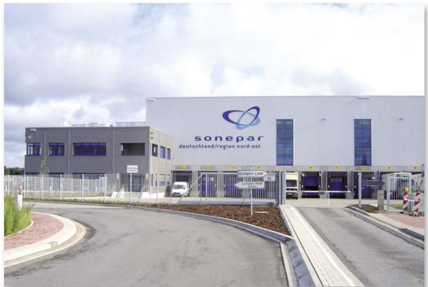
Sonepar-Zentrallager in Hannover.
